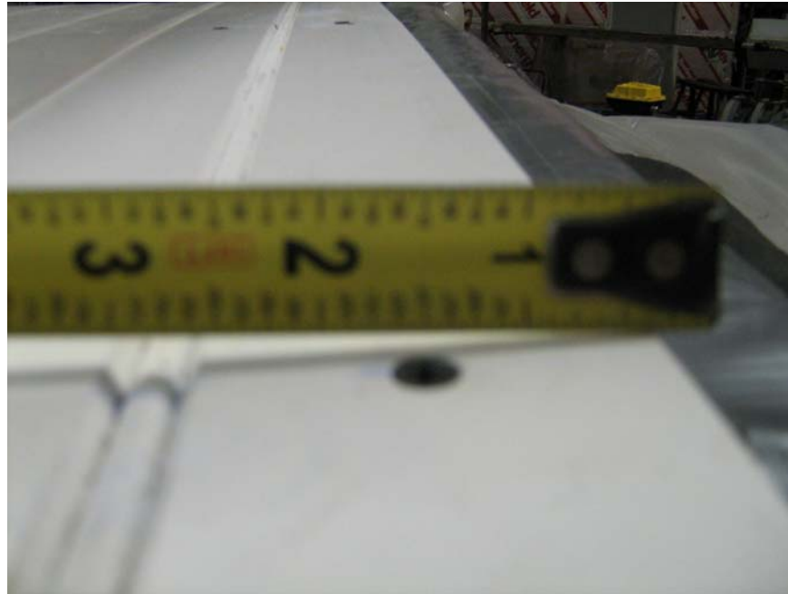
Photo No. 3 Installation
