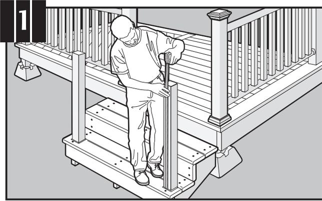
1 Measure post and cut sleeve 1" longer than post.
