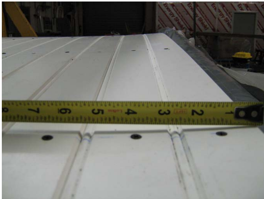
Photo No. 4 Installation
